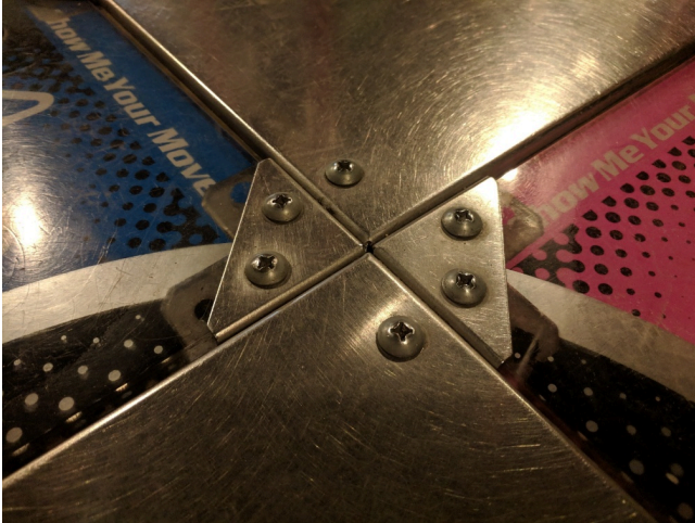
Figure 2. Detail of metal corner brackets, this paper’s namesake. Photo credit JIM.
